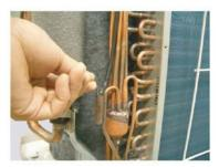
Remove the THERMISOTOR SPRING. Remove the THERMISOTOR.
