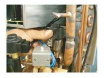
Remove the EEV coil by hand.
