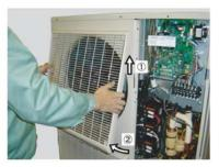
Remove the FAN GUARD by sliding upward.
