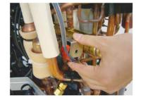
Remove the SOLENOID COIL.
