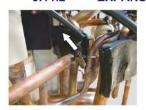
Remove the THERMISOTOR SPRING. Remove the THERMISOTOR.
