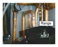
Cut the Discharge pipe in this range.
