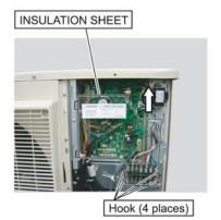
Remove the Hook. (4 places) Remove the INSULATION SHEET by sliding upward..
