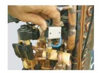
Remove the SOLENOID COIL.
