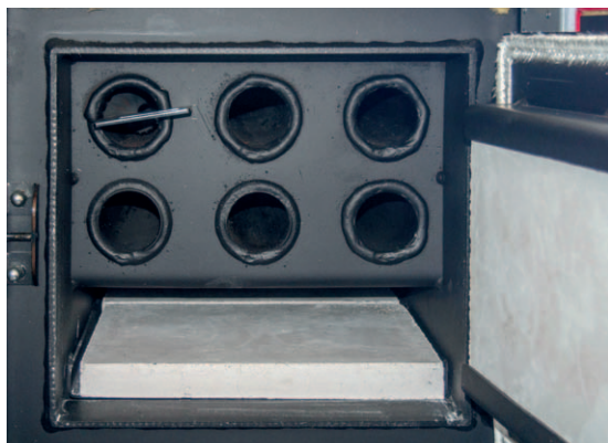
Detail of heat exchanger boiler A 15
