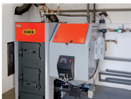
Model boiler room with boiler ROJEK TKA 25
