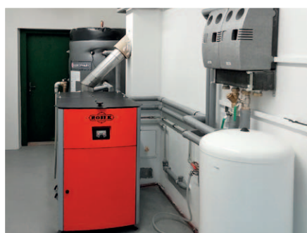
Model boiler room with boiler ROJEK PK BIO
